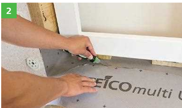
2 The windows are installed on the membrane. Before STEICOfix is installed, the sheet is cut back „half-moon-shaped“ (see Fig. 5).
