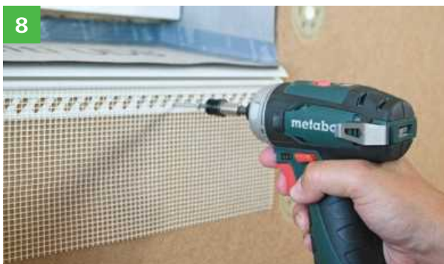
For a secure render connection, an attic profile is installed below the STEICO fix wood fibre insulation wedge (stainless steel screws or clamps in the wood fibre insulation board).
