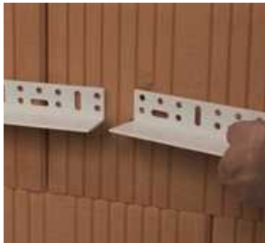
Attach angle rail
