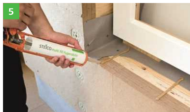
5 STEICOmulti fill adhesive beads are used to secure the insulation wedge against lifting off, e \leq 30 cm.
