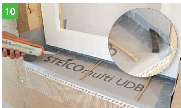
Application of STEICO multi fill adhesive beads e \leq 30 cm for the elastic fixing of the windowsill. TIP: Compriband strips glued at an angle guide any moisture that may enter safely to the drip edge.
