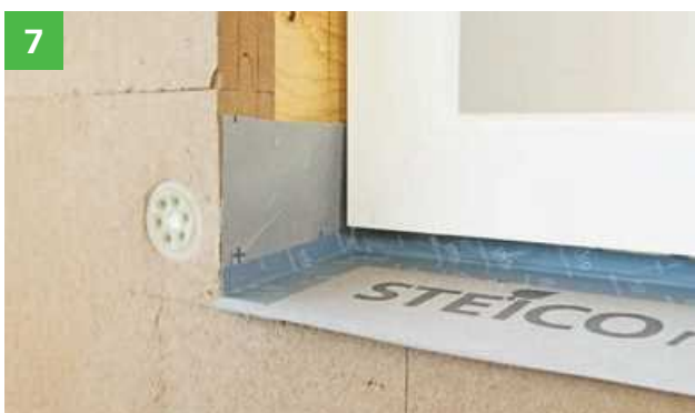
Insert the STEICO fix insulation wedge into the reveal, remove the remaining adhesive tape liner and press on the STEICO multi tape F adhesive tape.
