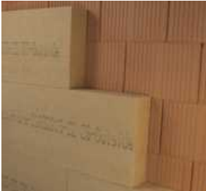
Installation of small-format square edge boards
